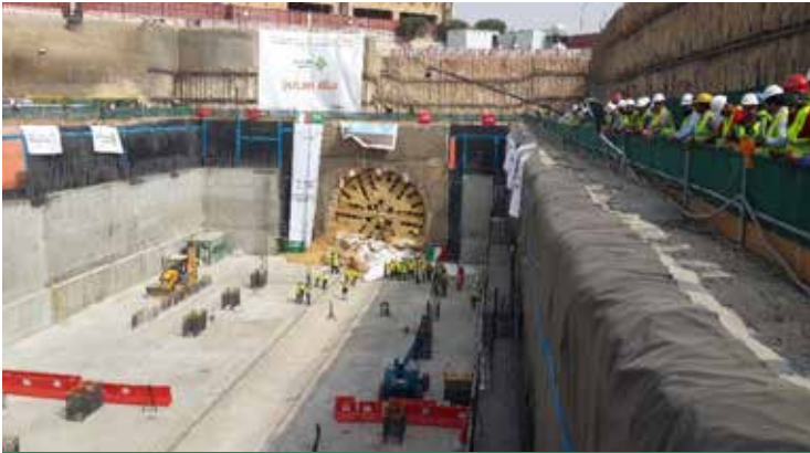
LINE 3 SHORING WORKS FOR THE TBM BREAK-IN BREAK-OUT
