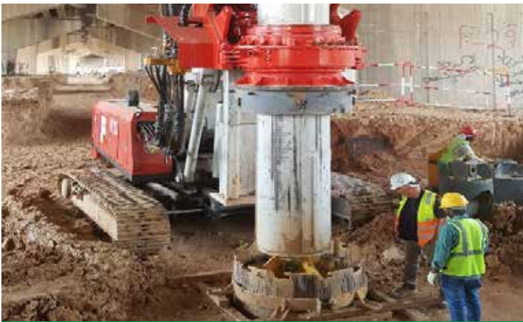
PILE DRILLING BELOW WADI HANIFA BRIDGE
